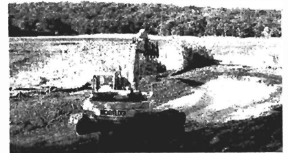
Stormwater basin under construction fall 2002.
