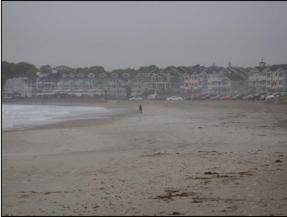
Figure 8. Seawall and low tide beach in front of the South Pavilion parking area (foreground of photograph).
