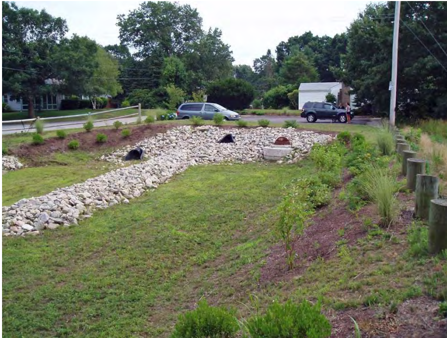
Mettatuxet Beach Stormwater BMP
