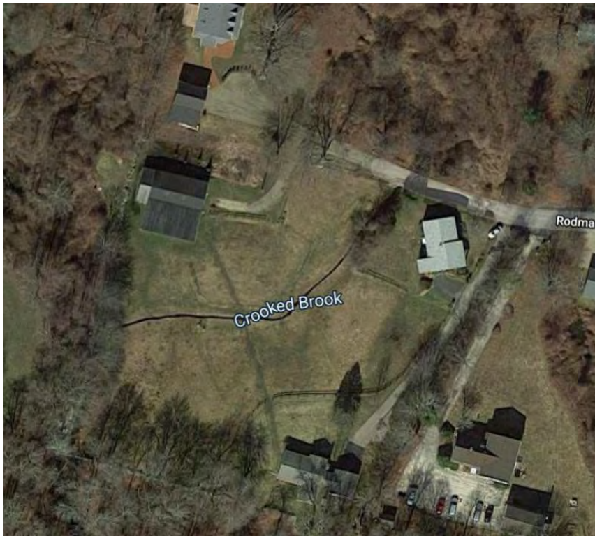
Example of missing buffer in the watershed to the Crooked Brook on private property. Google Imagery, 2019. (location: referred to as, 'horse farm property' in TMDL.)
