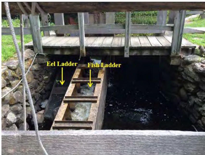
Picture of fish passages at Gilbert Stuart Museum dam. Image taken from Carr Pond Dam Visual Inspection/Evaluation Report by PARE Corporation, August 2014.
